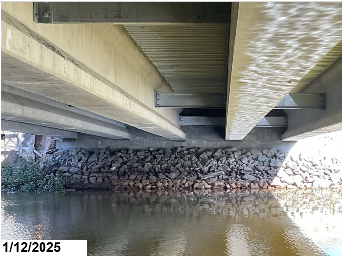
Bent 1: integral abutment overview.
