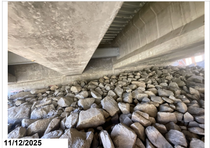
Bent 2: integral abutment overview.
