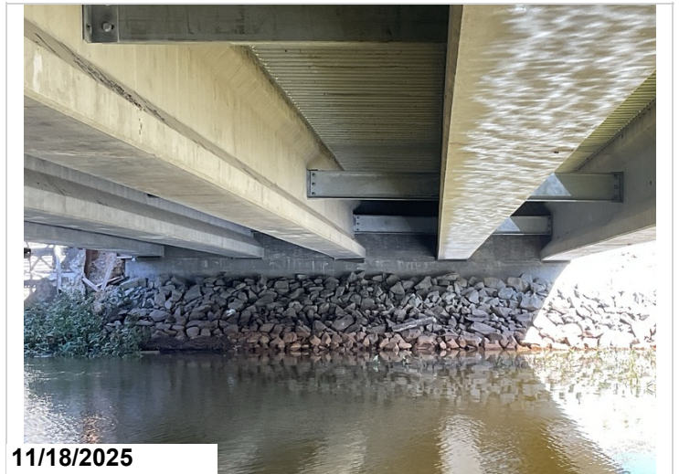
Bent 1: integral abutment overview.
